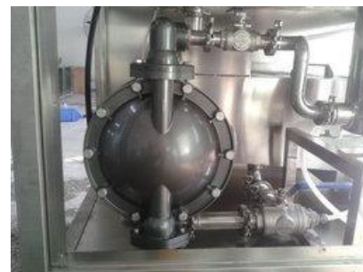
Pipe and Valve
