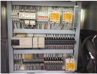
Control Box Mitsubishi,Schneider,CKD,Omron
